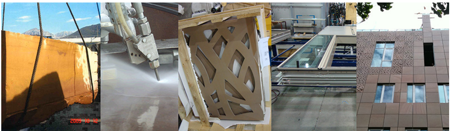
Figure 5. The offsite fabrication process for the unitized curtain wall system (from left to right): quartzite stone being quarried in northern India; water-jet cutting process in Carrara, Italy; finished laminated stone tiles crated and ready for shipment; assembling the unitized curtain wall sections in Montreal, Canada; craning the sections into place on the building façade in New York. Image courtesy of Machado and Silvetti Associates
